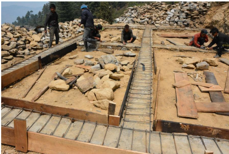
Wooden shuttering for the first seismic cement belt
