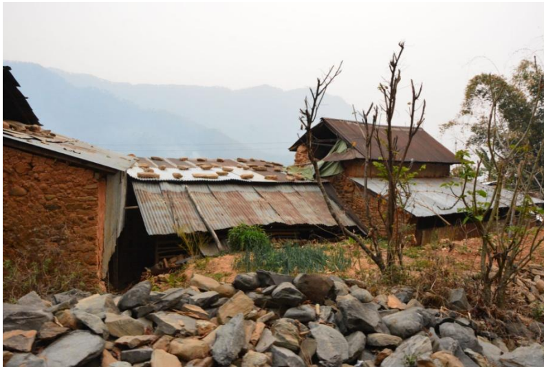
Destroyed houses provisionally repaired by corrugated metal
