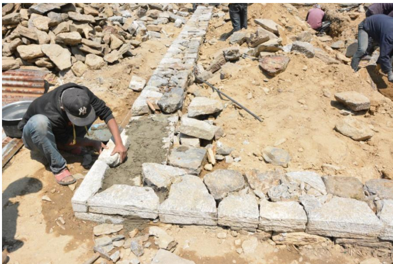
Fundament of the first model house in Brabal
