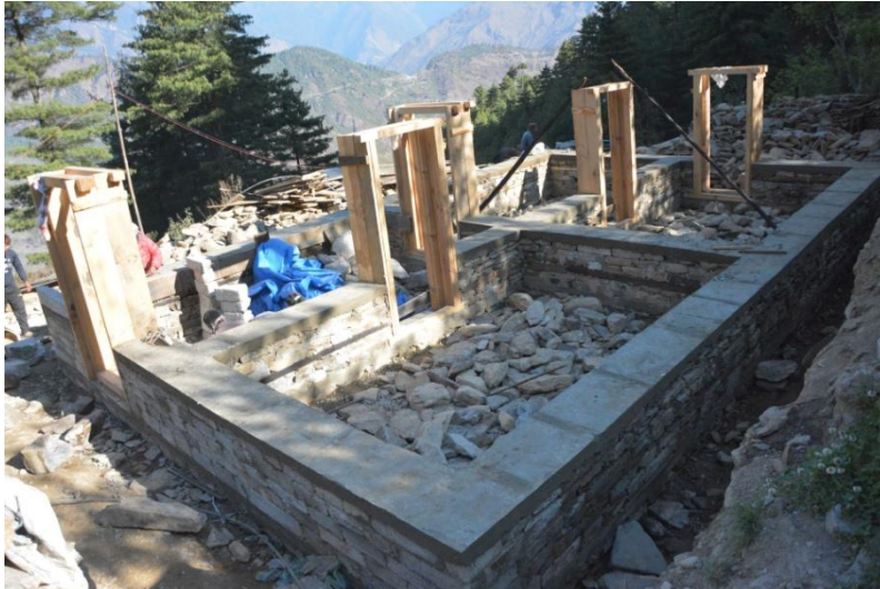
The doors are set
