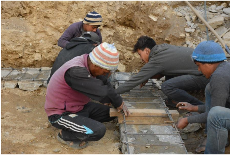
Iron hooks has to be placed exactly
