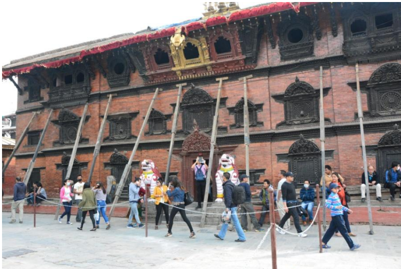
Kathmandu Durbar Square – Kumari-House with shoring
