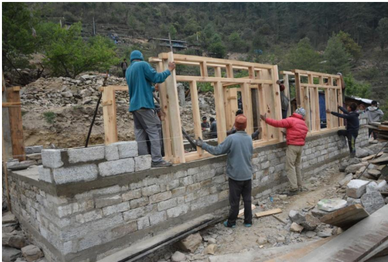
Construction's progress in Brabal – Installation of windows
